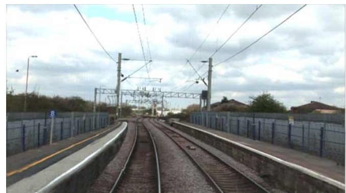
After Platform Extensions
