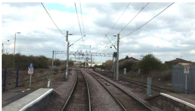
Before Platform Extensions
